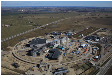
Aerial view of the ESS construction site, April 2020. Photo: Perry Nordeng
